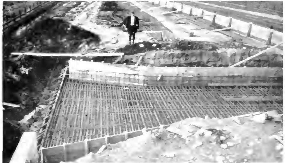
Fig. 43. Vallejo Creek. Construction of flare-siphon culvert
